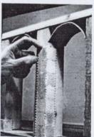
4. ADD FURTHER PAIRS OF PANELS IN THE SAME WAY UNTIL CLADDING REACHES TOP OF PIER, TAKING CARE TO KEEP EACH NEW PANEL FLUSH WITH THE LAST.
