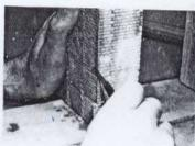
8. CUT OFF THE TWO REMAINING OVERLAPS, FLUSH WITH THE LINKA SURFACE.
