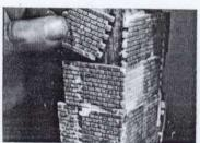
7. STARTING AT THE OPPOSITE CORNER, REPEAT PROCESS UNTIL THE ENTIRE PIER IS LINKA CLAD.
