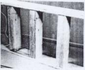
BUILD A WOODEN FRAME -WORK. (The bottom strip can be a temporary keep to hold the piers square during construction.)
