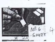
ETCH IN MORTAR LINES ON SANDED AREA.
